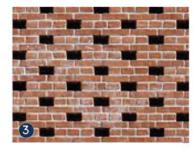
Perforated Intake / Exhaust Brickwork
